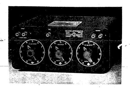
The Type 1450 Decade Attenuators are precision adjustable attenuators designed for use either in balanced H or unbalanced T-type 600-ohm circuits. They are especially useful for precise power level measurements, transmission efficiency tests, gain or loss measurements on transformers, filters, amplifiers and similar equipment, and for calibrating other attenuators. Each type is available in two- or three-decade ranges as follows:
